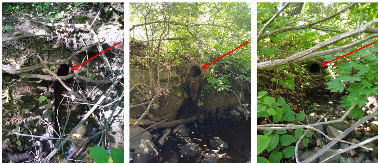
Figure 6: Pipes with elevated detergent levels. Left to right: AS-03, AS-08, AS-09. AS-03 had very high levels – located river right facing downstream near the middle of the parking lot for 50 Main Street.
