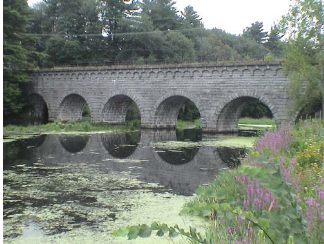
MDC Aqueduct Upstream of Assabet River Dam
