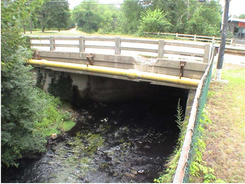
Route 20 Bridge Just Downstream of Dam
