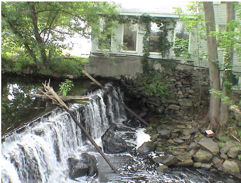
Dam and Left Abutment
