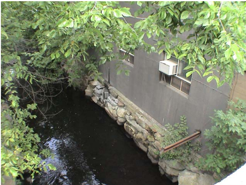
Support Walls Just Downstream of Route 20 Bridge
