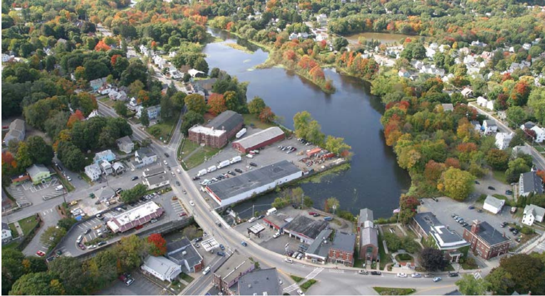
Aerial Photograph of Hudson Dam
