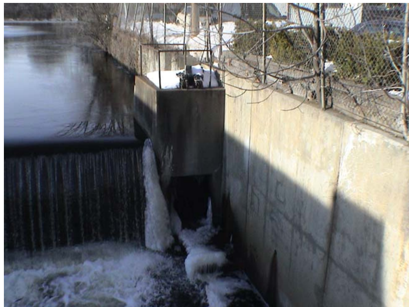
Gated Outlet Works for Hudson Dam
