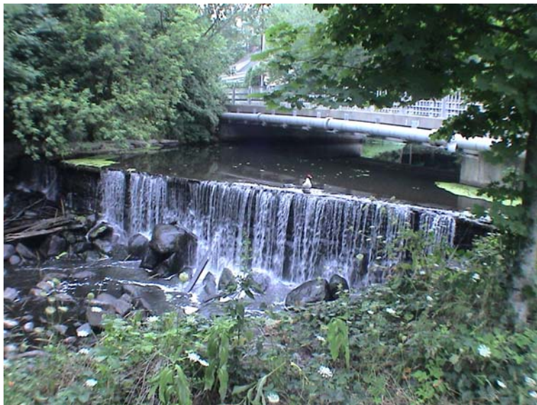
Allen Street Dam
