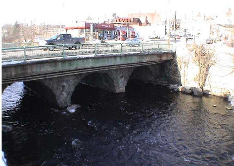
Hudson Bridge and Old Arch Stone Culvert Bridge
