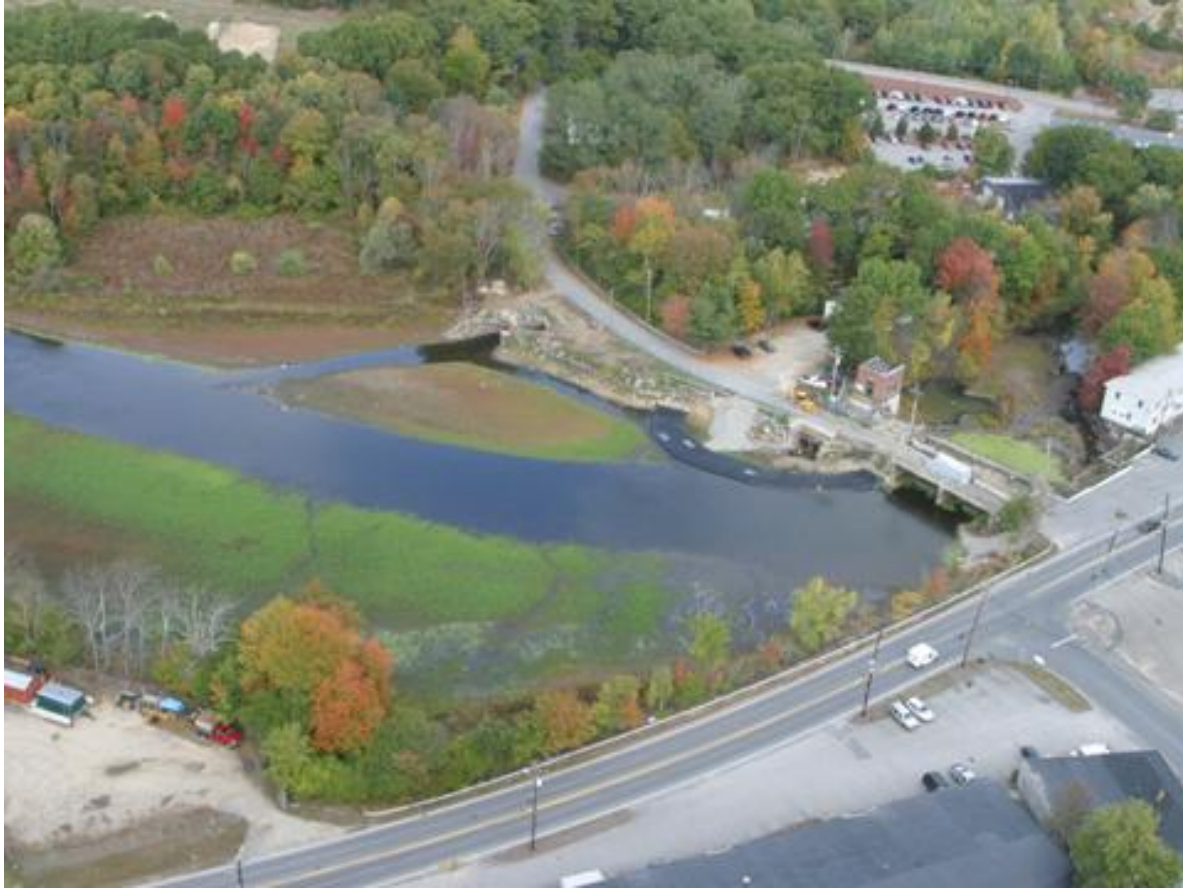
Aerial view of dam prior to reconstruction
