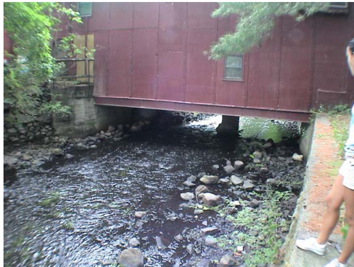
Apartment Unit Walkway Downstream of Assabet River Dam
