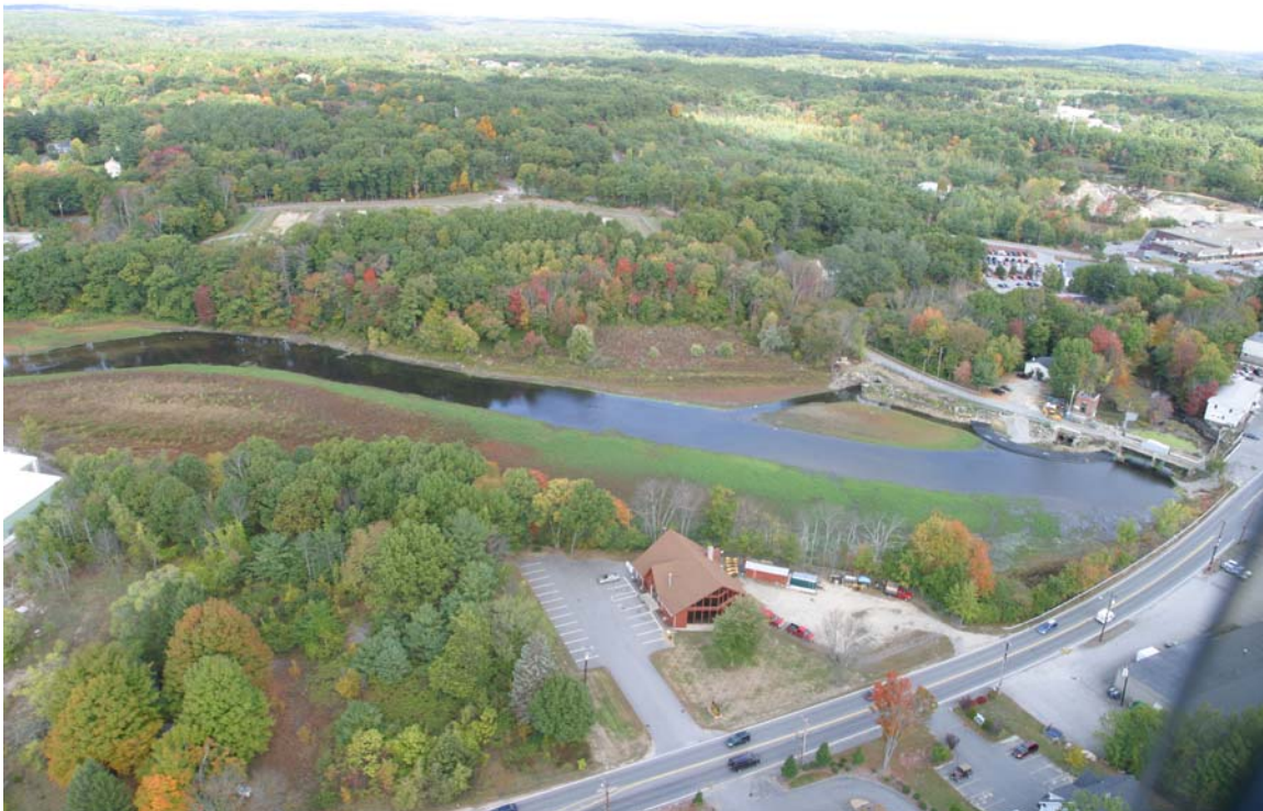
Aerial showing lower impoundment level due to extended drawdown
