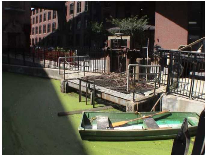
Hydropower Intakes at Mill Complex
