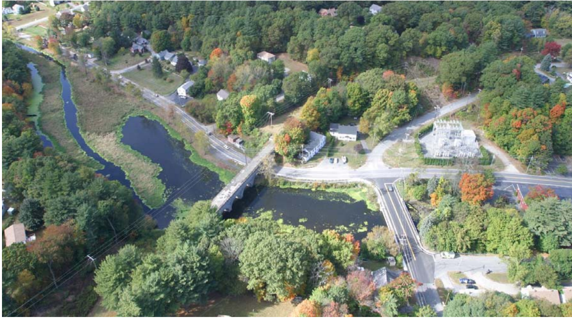
Allen Street Dam Impoundment
