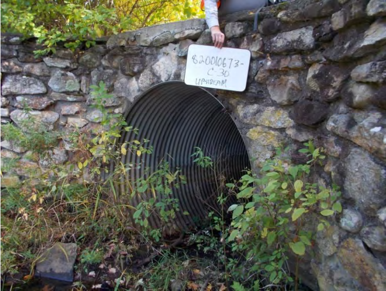
Culvert at Vega and Goodale Roads, Marlborough
