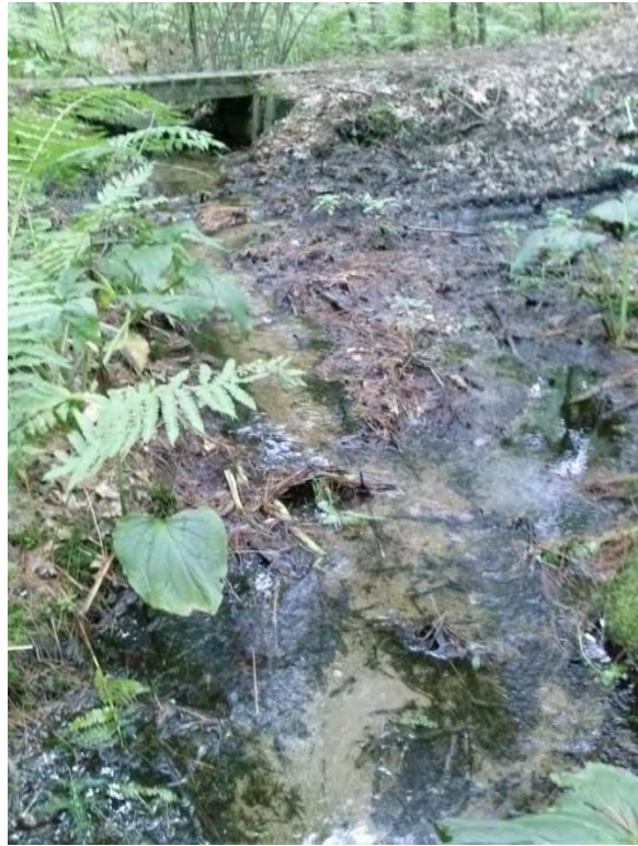
Figure 4: Erosion at unnamed tributary
